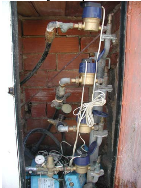
Figure 9. Precision water meters and data-loggers used for the study
